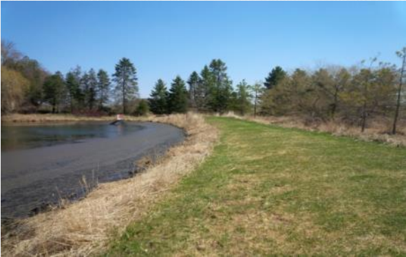
Low earth fill embankment, a grassed, emergency spillway is located at the east end of the embankment. This spillway has a clear width of about 4.0 m and the inlet invert is 0.6 m below the crest of the dam.
