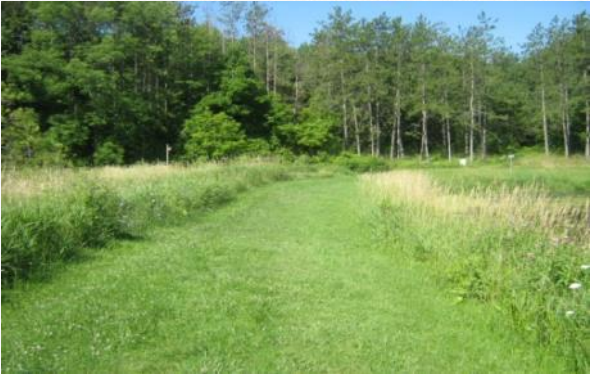
The Embro Dam is approximately 100 m in length, 4.5 m in height and includes 1.1 m of freeboard. The entire dam is founded on overburden as opposed to bedrock or engineered soil.
