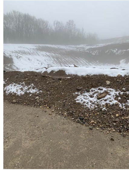
2020/11/26 07:49:55 Rehab-LookingSouthwest.JPEG Taken by: Steve Oliver
