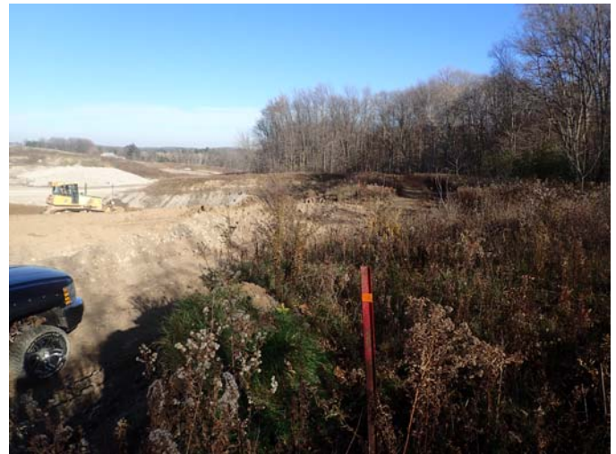
2020/11/09 13:59:50 TG-4;PB090116.JPEG Taken by: Stephen Douglas Setbacks along the woodlot that occurs along the S part of the site is well-marked with red-painted t-bar posts
