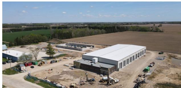
Late in 2020, Council approved construction of the Zorra Maintenance Facility at a cost \$10 million. This facility will be carbon neutral, solar powered and heated and cooled using a geothermal HVAC system. In evaluating options for this building, Council reviewed 50-year life cycle costs and determined the most efficient option was go completely carbon neutral.
