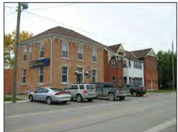
Commercial Uses on Huron Street
