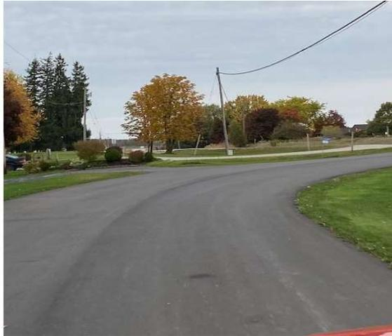
★ Completion of Road 98: pulverized & pave with culvert replacement. Second layer of pavement to be completed in 2024.
